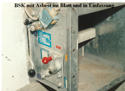
Fire protection flap with asbestos in the flap and in the frame
