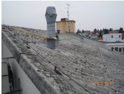
Asbestos cement roofing
